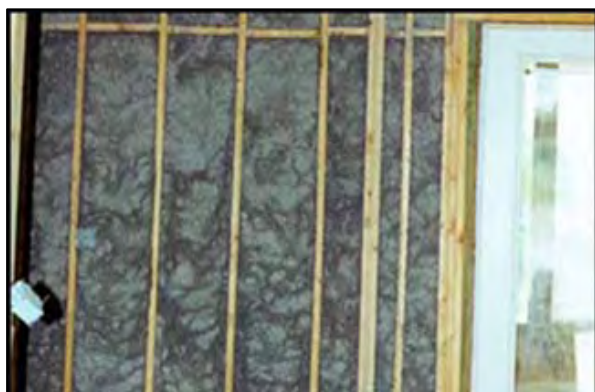
Basement wall insulation
